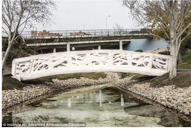
Figura 27. Bridge built through 3D printing in Spain (dailymail.co.uk)
