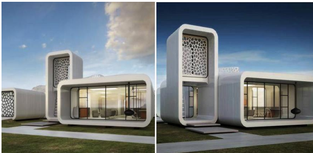
Figura 26. Building constructed by 3D printing in Dubai (3dprint.com)
