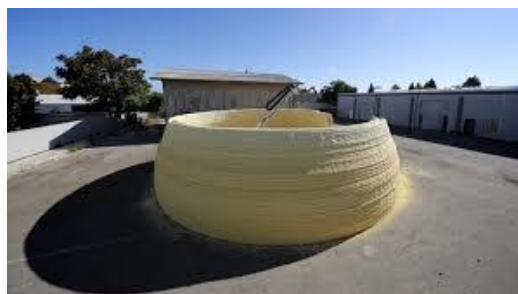
Figura 25. Prototype created by DCM, it is a dome 50 feet in diameter and 12 feet high ( money.cnn.com/2017/05/02/technology/3d-printed-building-mit/ )
